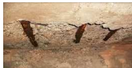
Fig.34 corrosion on concrete
